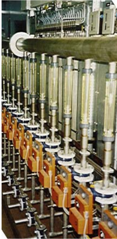
Figure 18. The typical manifold in Nordic countries. Automated volume control and rotameters for manual volume registration on each well. Denmark.
