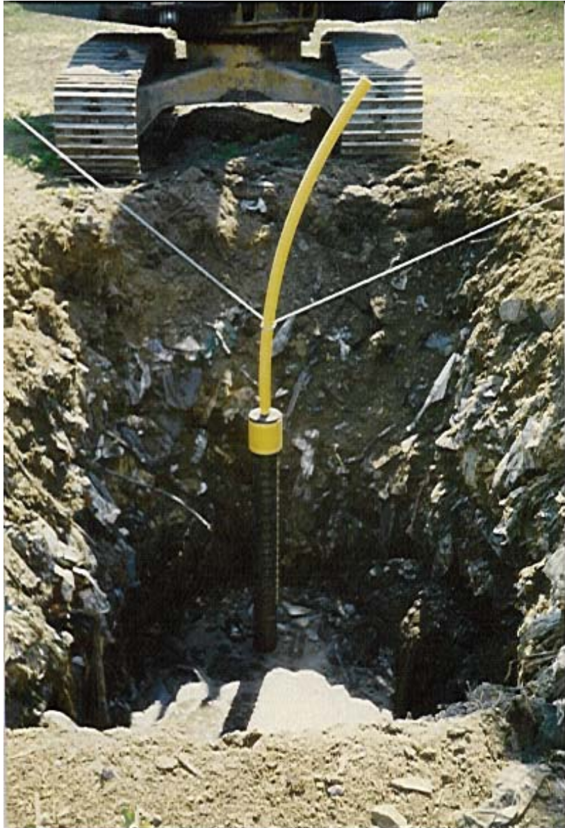
Figure 7. Large size well – diameter 1500 mm (Kastet – Norway)
