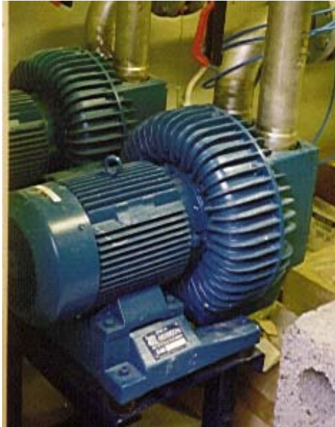
Figure 15. Side channel blowers are common to create an underpressure in Nordic LFG plants (Fitjar, Norway)
