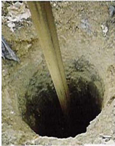
Figure 8. Large size well – diameter 600 mm (Gatedalen, Norway)
