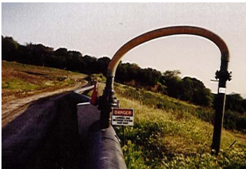
Figure 10. In the US pipelines are located on the ground and the wells are connected directly to the pipeline in open air (Orlando landfill, LA)
